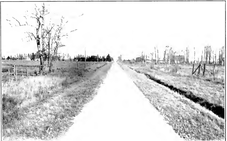
Typical Township Road.
